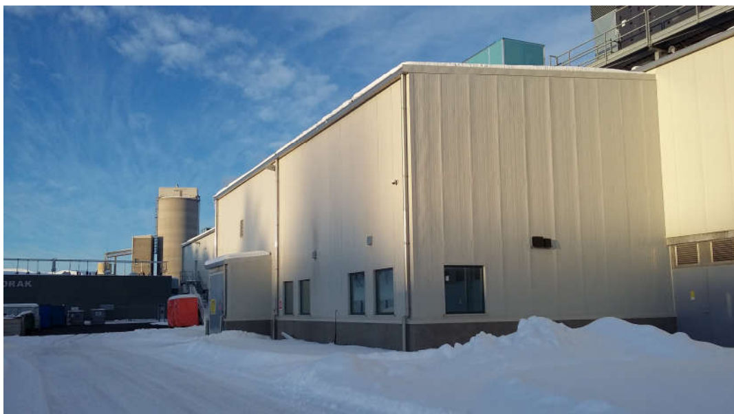
Figure 5: Second measurement location.
